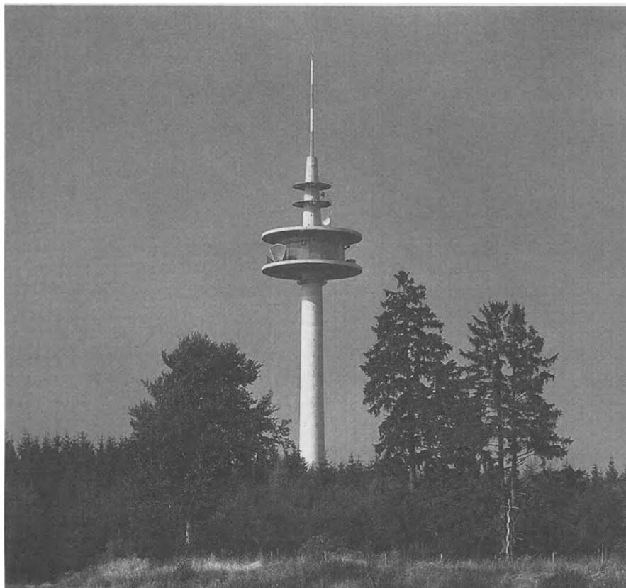
Fig. 16.1. Telecommunications tower. (Photo by courtesy of Siemens AG)
