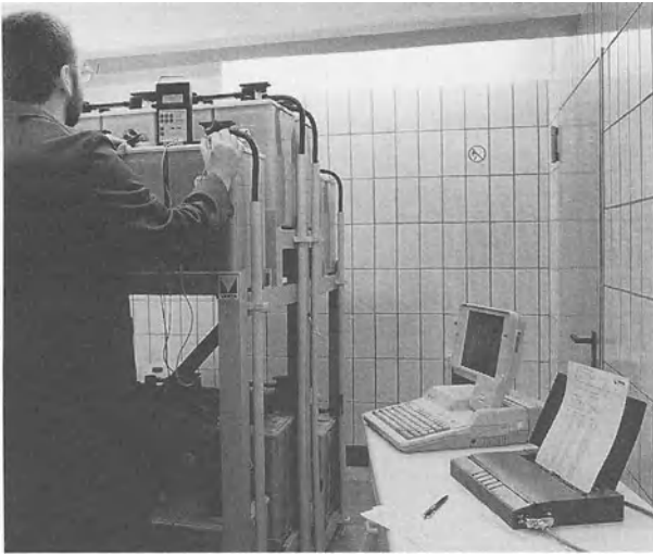
Fig. 6.22. Measuring and testing of a battery system for UPS. (Photo by courtesy of Varta AG)
