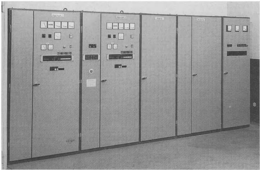
Fig. 15.4a. Control cubicle for fully automatic alternating operation. (Photo by courtesy of AD. Strüver KG, GmbH & Co.)
